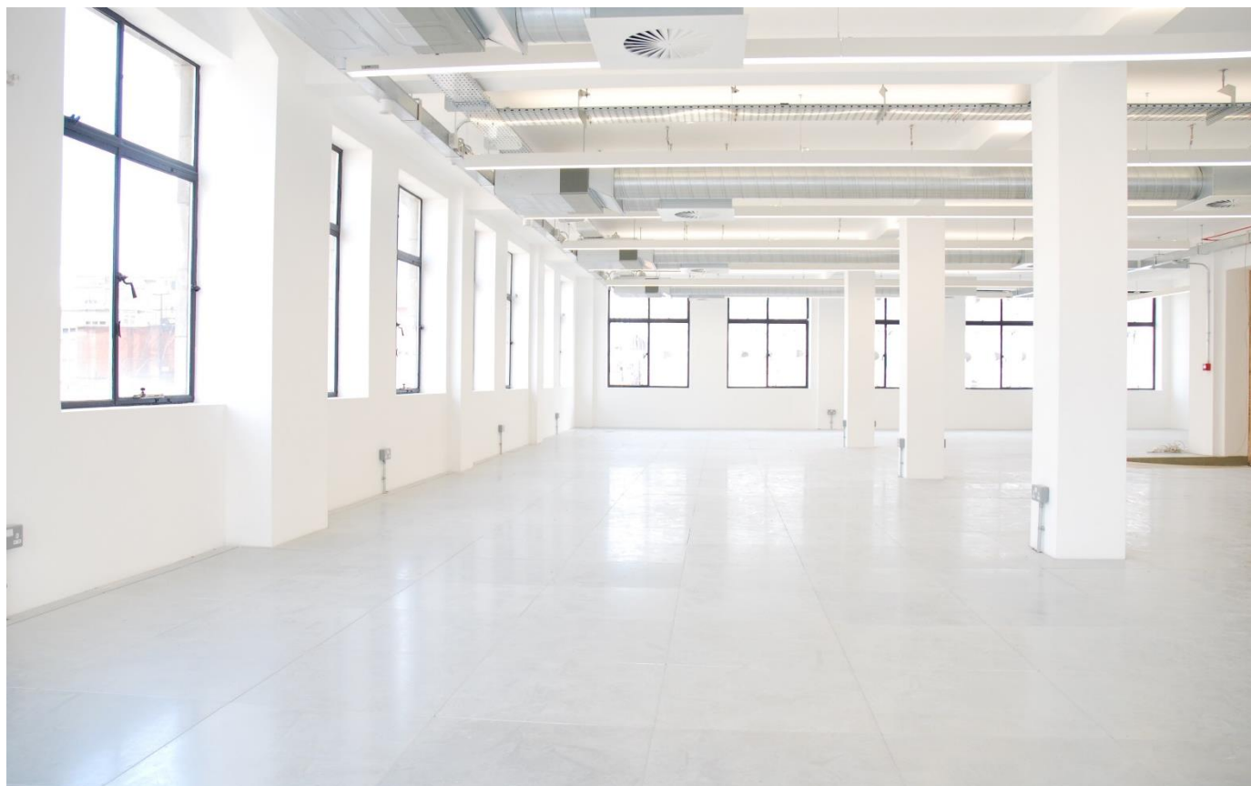
Refurbished 4th floor north
